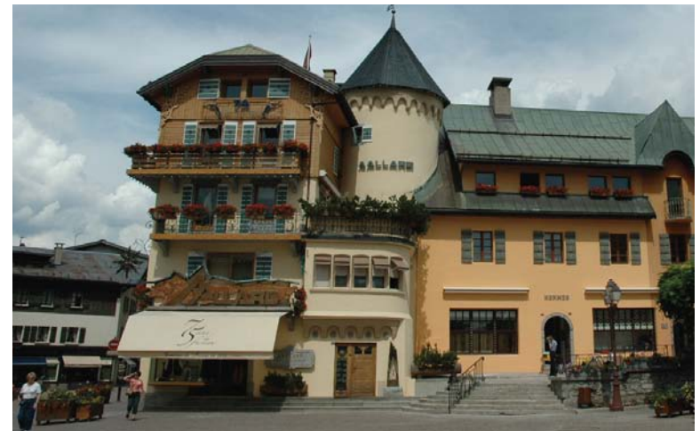
Fig. 1: A vibrant village with varied building forms and asymmetrical window patterns.
