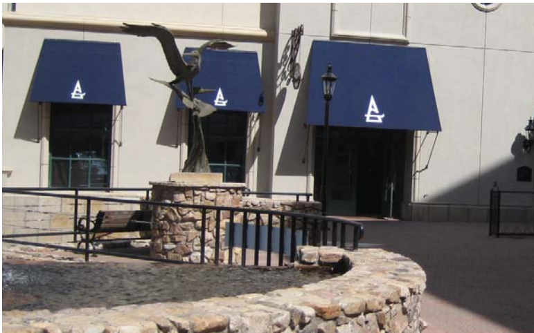
Fig. 5: Canopies add color and shade protection to the building
