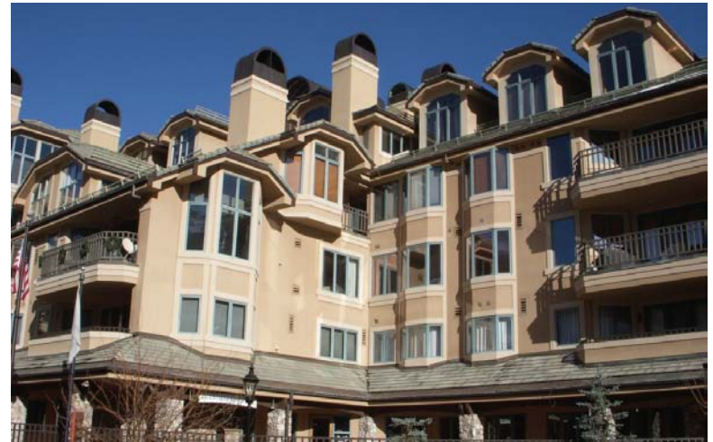
Fig. 2: Chimneys and Roof vents
