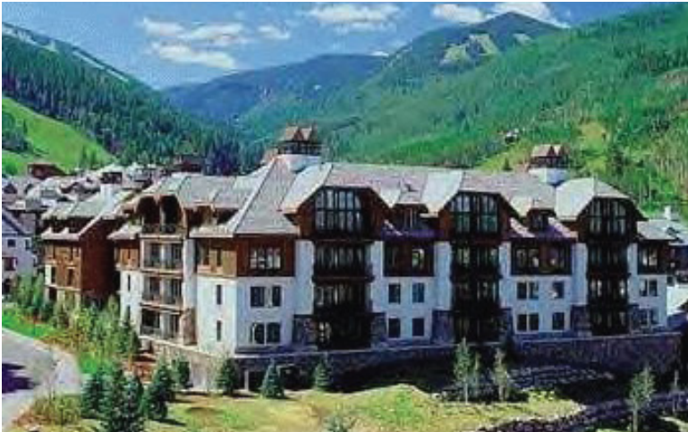
Fig. 5: Exterior building materials (stone, stucco and wood siding)
