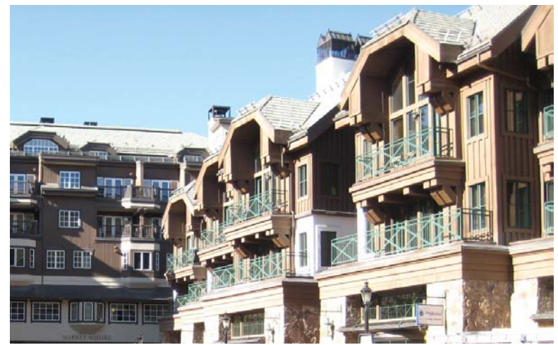
Fig. 1: Exterior building materials (stone, stucco and wood siding)
